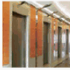
Multiple Elevators per Building
